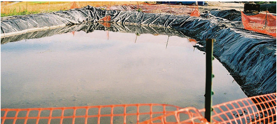
Silpaulin water storage tank
