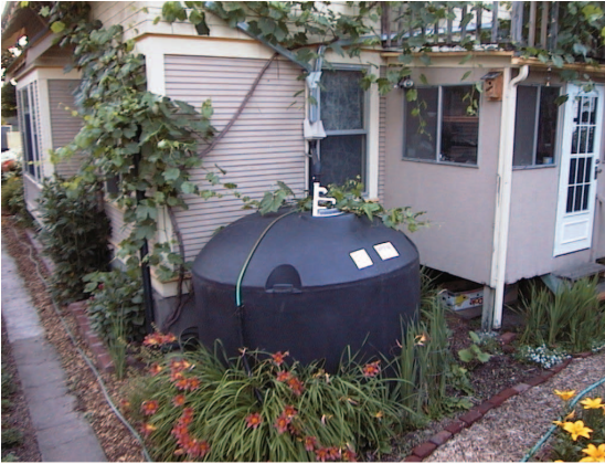
Rain water storage tank
